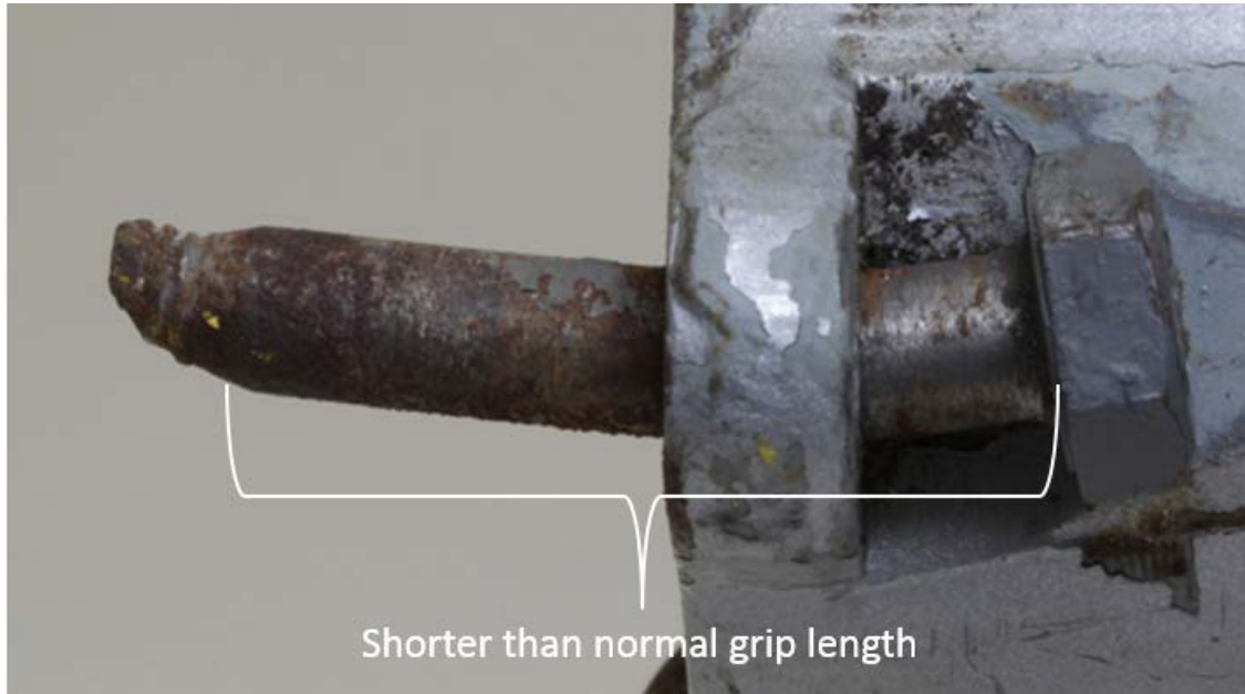
Figure 30: One of the non-standard upper attachment bolts fitted to VH-TSG showing the shorter-than-normal grip length
